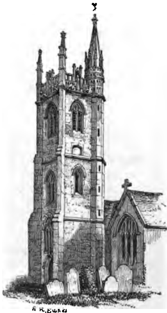
156. Brislington, Somersetshire, c. 1500. Shewing the diagonal corner buttresses and stair-turret, with the open parapet and pinnacles.
